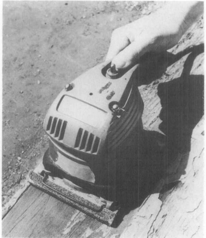
Fig. 11 The orbital sander can be used for limited paint removal, i.e., for smoothing flat surfaces after the majority of deteriorated paint has already been scraped off. Photo: Charles E. Fisher, III.
