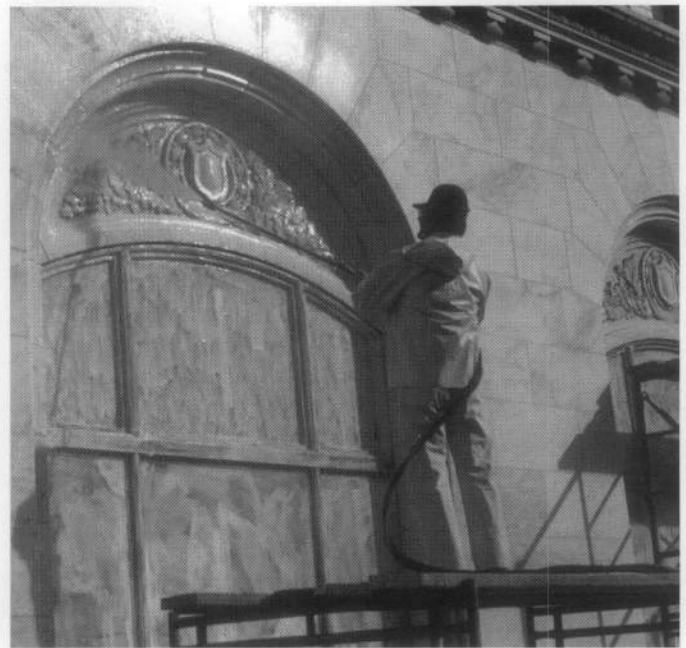
Figure 7. Glazed architectural terra cotta often may be cleaned successfully with a low-pressure water wash and hand scrubbing supplemented, if necessary, with a non-ionic detergent. Photo: National Park Service Files.
