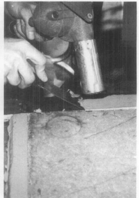
Figure 4c. Sash can be removed and repaired in a convenient work area. Paint is being removed from this sash with a hot air gun while an asbestos sheet protects the glass from sudden temperature change. Photo: John H. Myers
